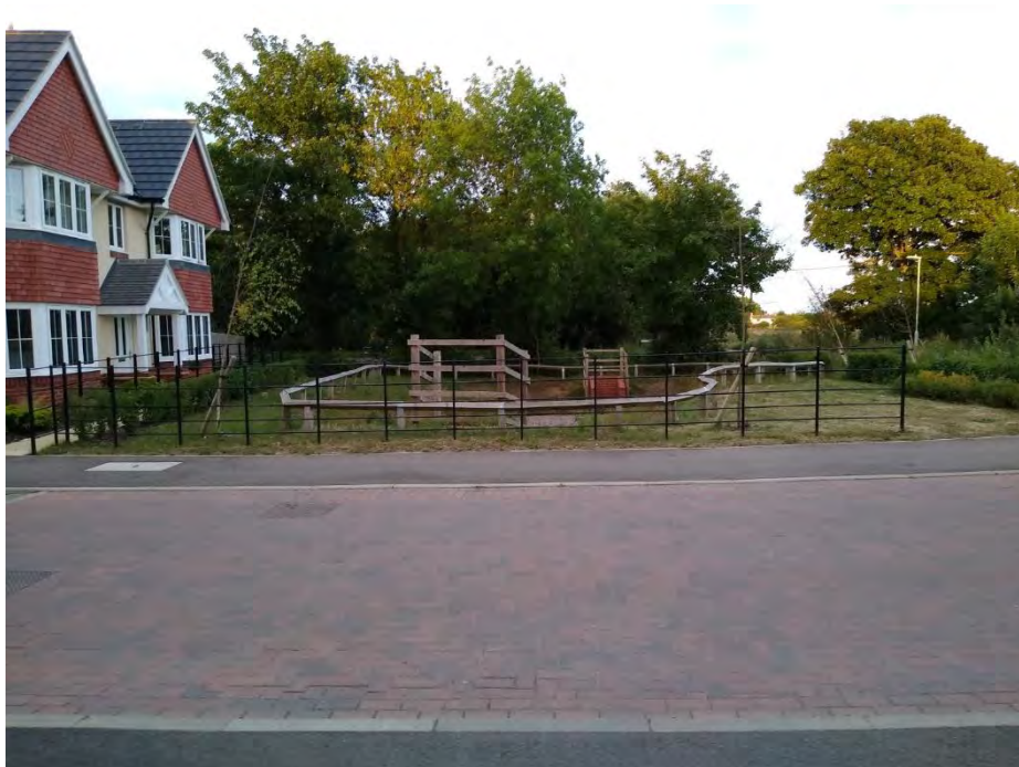
Figure 6.10: Fencing surrounding drainage basin created as part of new development along Bannold Road
